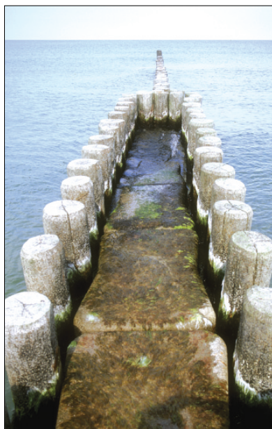
Abb. 5: Kastenbuhne in Abrenshoop/ Fischland; Box-shaped groynes at Abrenshoop/ Fischland. Foto: Archiv IWR
