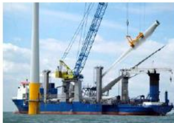
Leg-stabilised crane vessel
